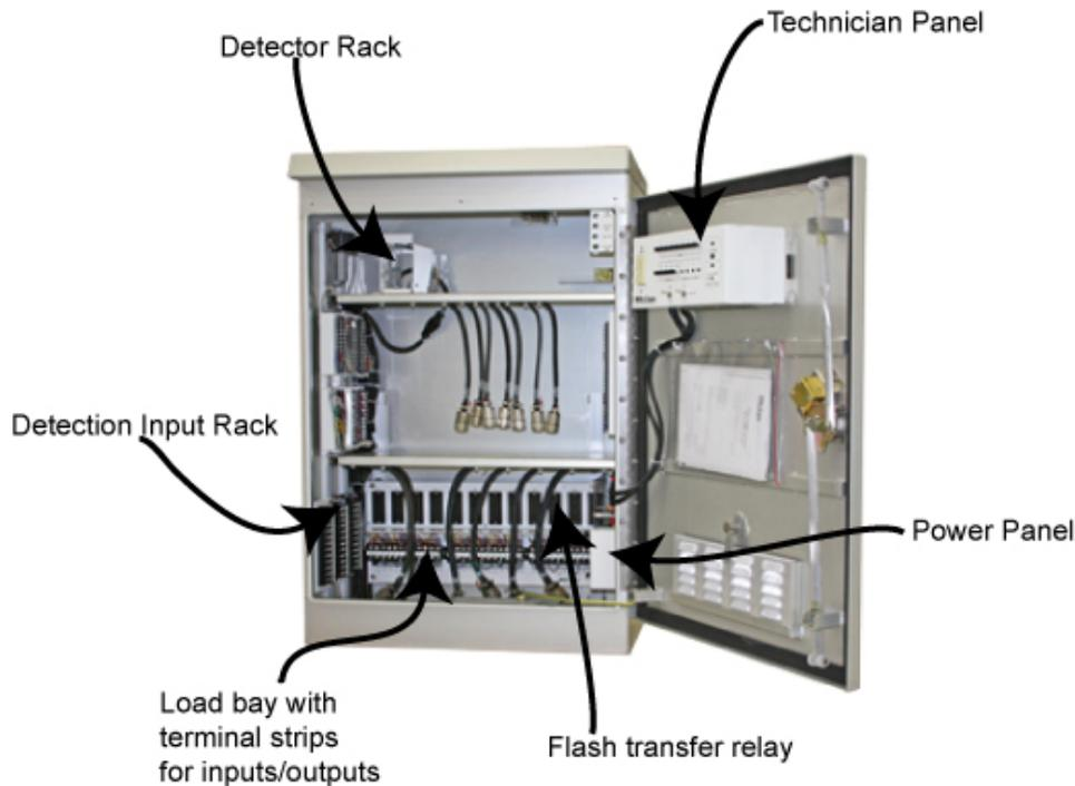
Inductive loop detections plug into the detector rack at the top of the controller. When you order a cabinet, you don't get the loop detectors, you just get the rack.
